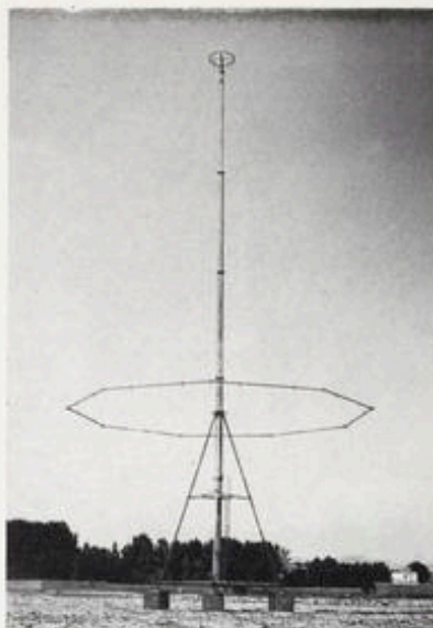
The 31-metre high circular aerial for the short wave transmitter
